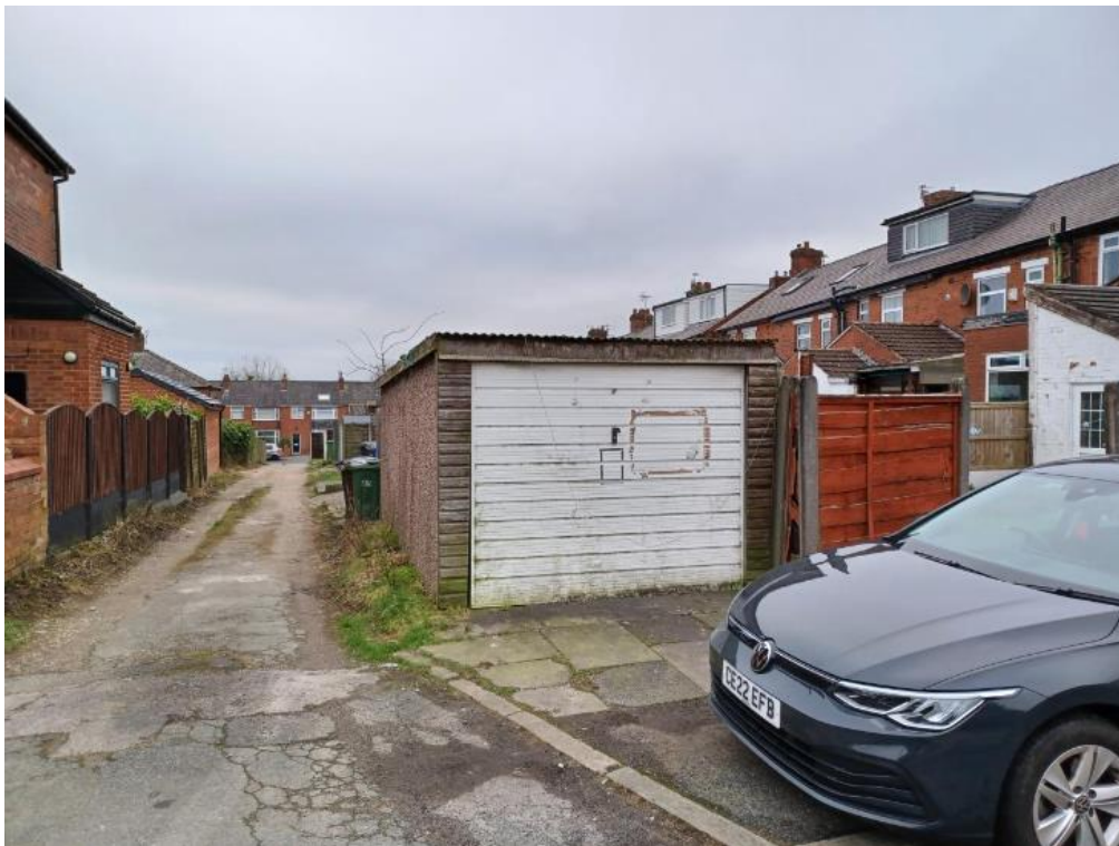
Photo 4: Existing garage, to be demolished, to provide 1no off street parking space, access taken from Bedford Avenue.
